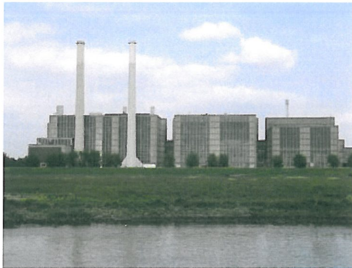
IJsselcentrale, rivierzijde (west) in 2012
